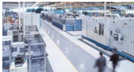
Polpenazze production facility - Italy
